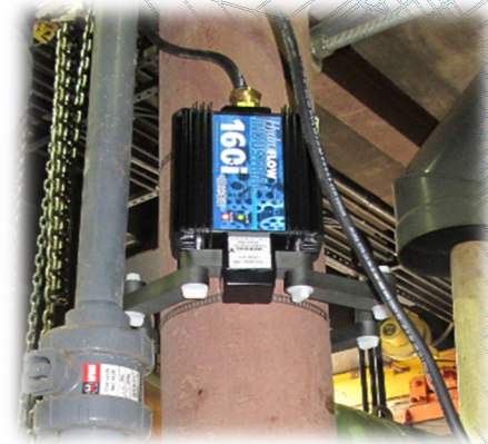
Mounted on a 6 1/2" line for a belt filter press for struvite scale reduction, Wastewater Treatment facility Rockland County, NY
