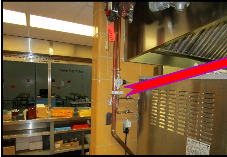
HydroFLOW S38 installed on cold water supply line feeding the steamer oven
